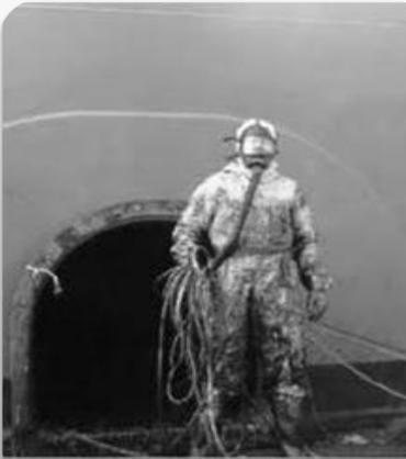
**Manual Cleaning:** This involves entering the tank and using manual labour to remove the sludge. It is usually done in teams because of the potentially hazardous chemicals that are found in sludge. Persons involved in manual cleaning of these oil tanks are also equipped with Personal Protective Equipment (PPE)
